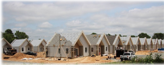
Serenity Courtyard of Macon construction site
