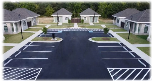
Photo courtesy of Stafford Builders & Consultants, Inc. of Completed Tiny Cottages of Macon
